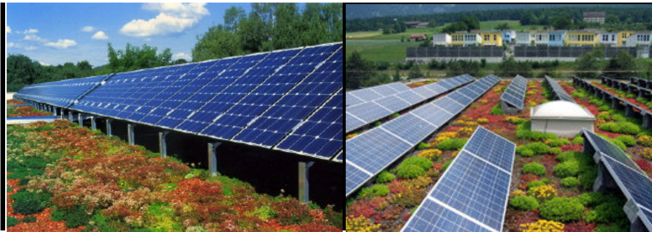
Figure 7.1 PV integrated onto green roof
