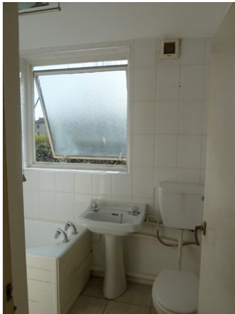
Fig.10 The current bathroom within the rear extension – note the aluminium window to be replaced with a glazed timber door and casement under the retained lintel.
