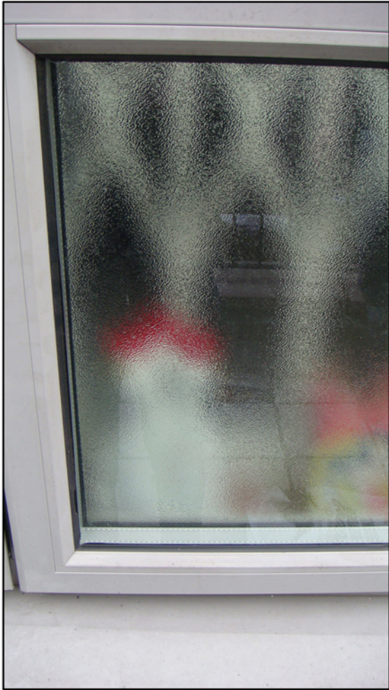
Second level windows - Obscure glazing
