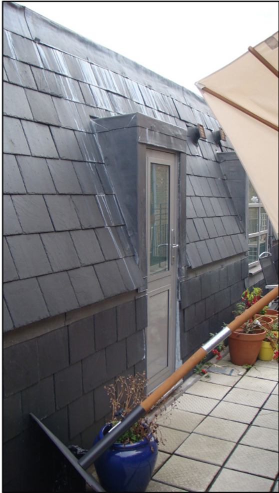
Second level door onto the rooftop
