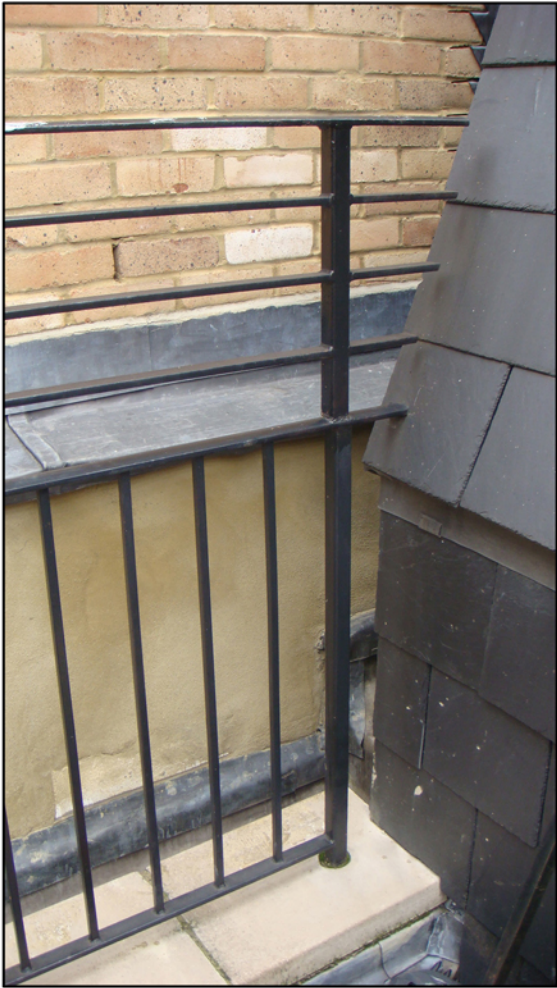
Second level handrail - Joint with mansard roof
