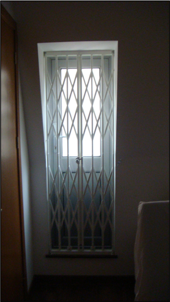
Second level door
