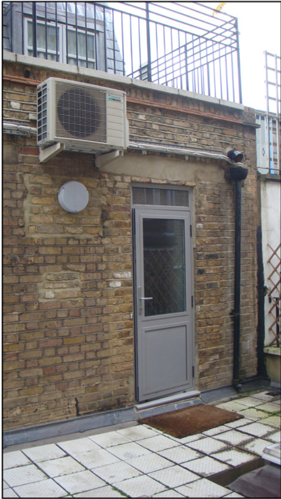
First level door onto the rooftop
