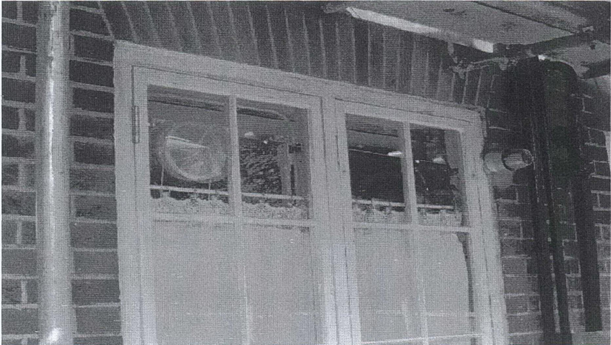
Kitchen window of 112 Croftdown Road (Rear Elevation). Window in timber single glazed.
