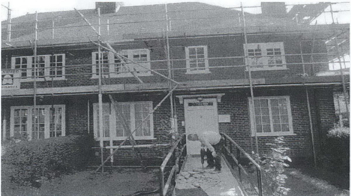
Front Elevation. 112 Croftdown Road on Ground Floor with timber single glazed windows and 114 Croftdown Road on Ground Floor with timber double glazed windows and 110 and 116 Croftdown Road on First Floor with timber double glazed windows.
