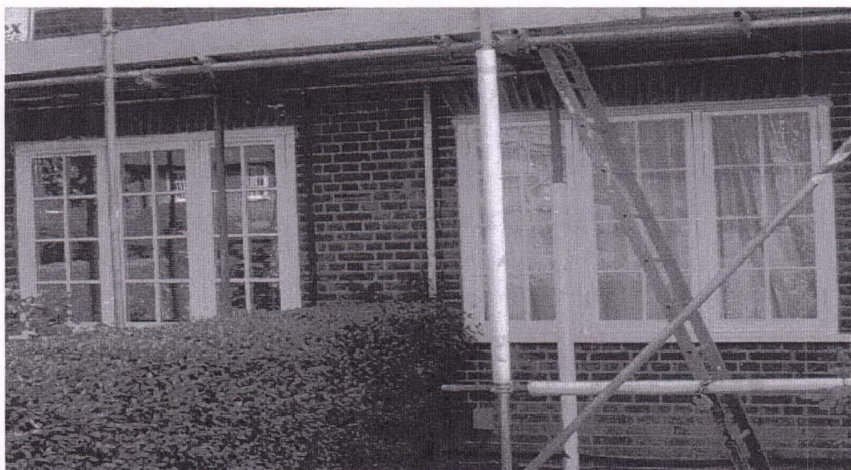
Sitting Room windows at Ground Floor (Front Elevation). On the right hand side the 112 CR with timber single glazed windows and on the left hand side 114 CR with timber double glazed windows.
