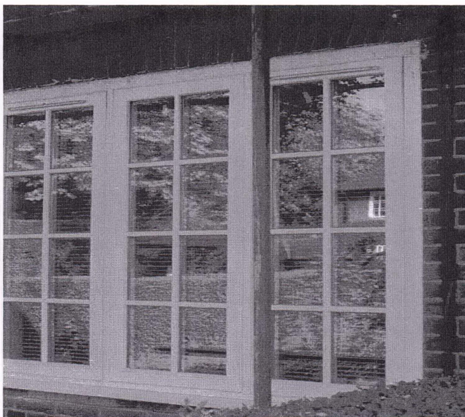
Sitting Room window at Ground Floor (Front Elevation). 114 Croftdown Road with timber double glazed window.
