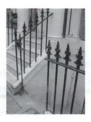
Example of similar stair layout at No 11 Chamberlain Street – Proposed stair will be constructed of stone treads on a concrete base with a metal railing balustrade to both sides and a lockable gate installed within the existing metal railings at pavement level that will be made out of the section of railings that will create the access.
