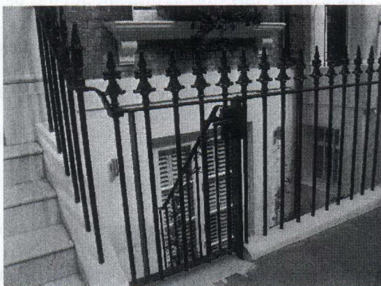
Railings to basement area. No. 11 Chamberlain Street (left) and No. 12 (right). The retention of the base plinth would help to minimise the impact of inserting a gate.
