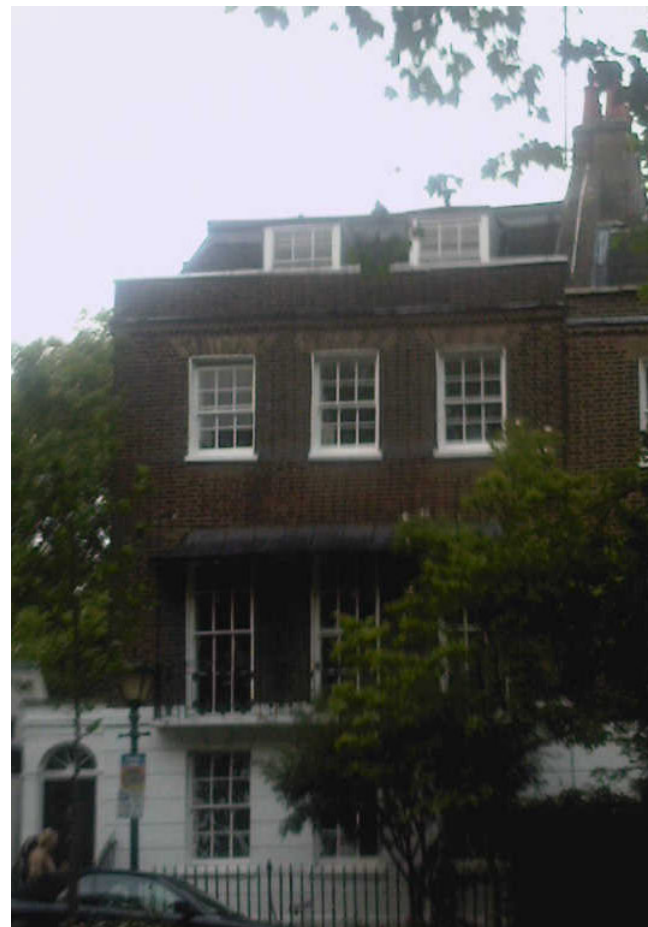
Raised coping detail to the front of the windows to lessen impact of Mansard
