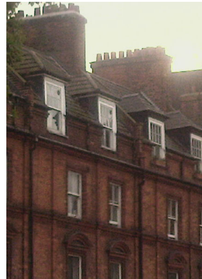
Raised coping detail incorporated with the mansard roof windows emphasises the height of the building.
