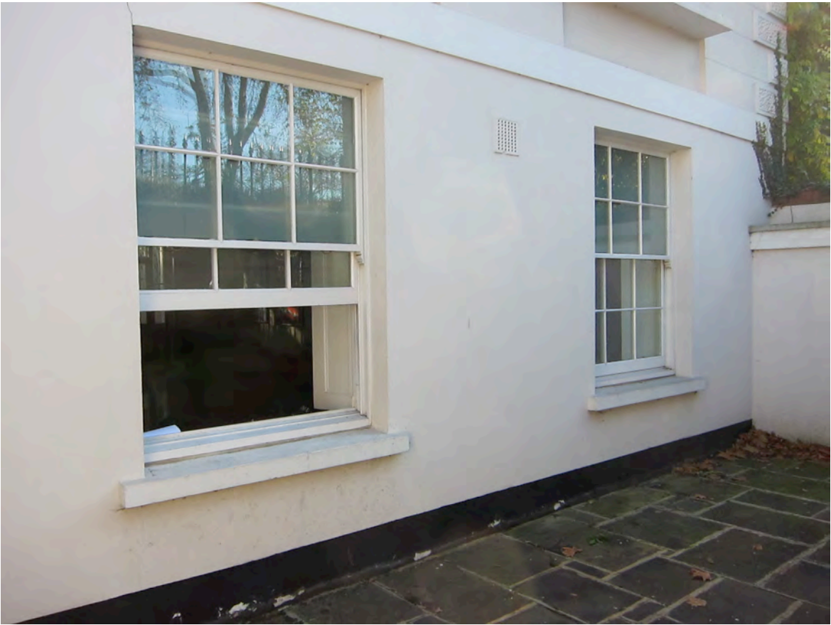
1 Existing Timber Sash Windows
