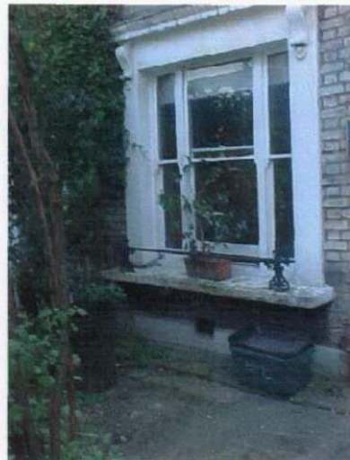
GROUND FLOOR WINDOW No 7
