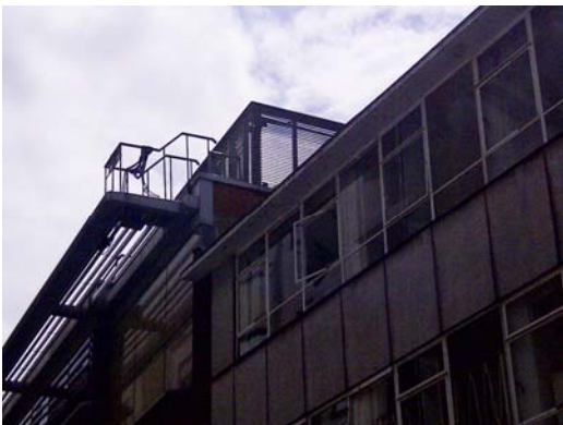
No. 91-94 Saffron Hill with visible rooftop louvered plant enclosure
