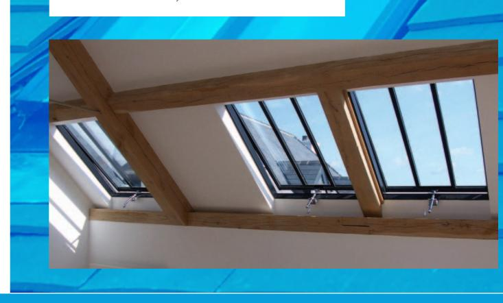
We also offer the Lumen Conservation rooflight in bespoke sizes and designs. Conservation organisations stipulate that the minimum amount of framework should be visible and this requirement becomes even more significant when rooflights are placed next to each other.
