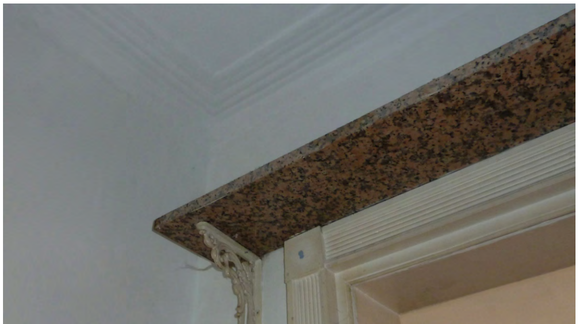
Appendix 2: 2.30 Detail of the modern door surround and original cornice at the ground floor rear room.
