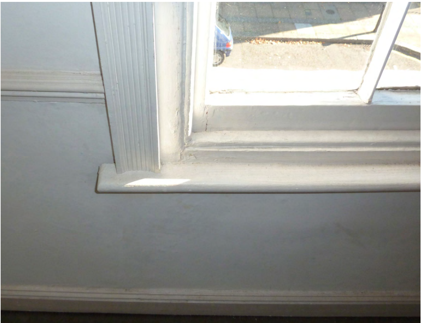
Appendix 2: 2.46 Detail of an original window with modern surround at the second floor front room.
