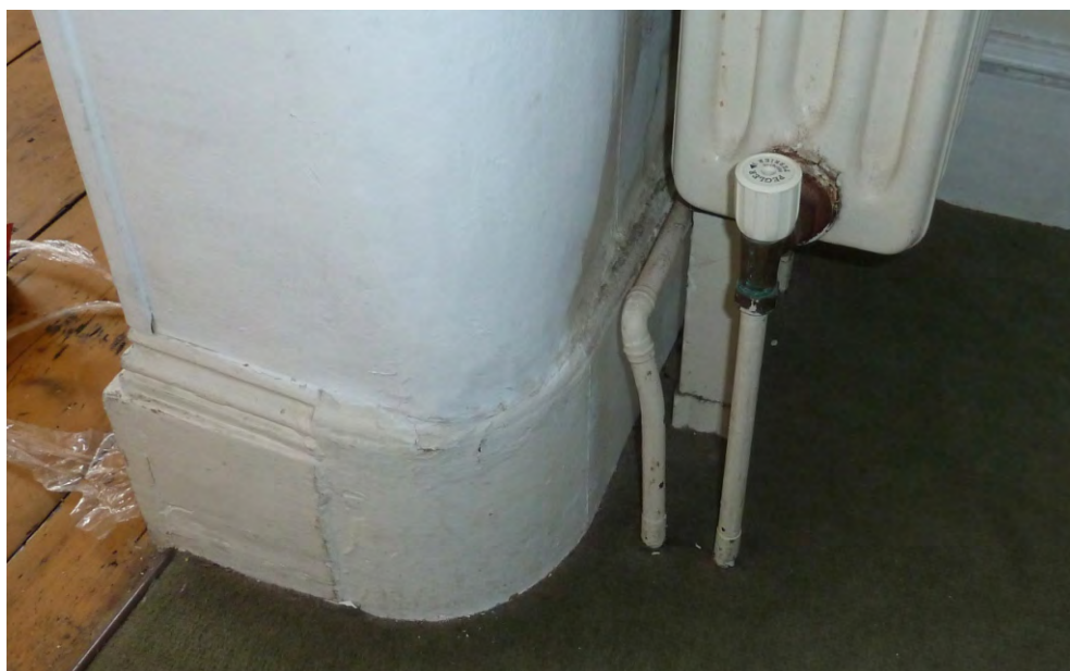
Appendix 2: 2.33 Detail of original skirting at the curved stairwell corner.
