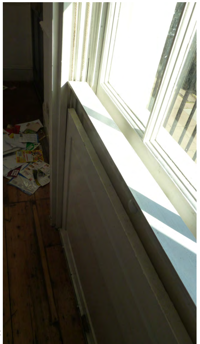
Appendix 2: 2.28 Detail of the window and the vertical sliding shutter at the ground floor front room.
