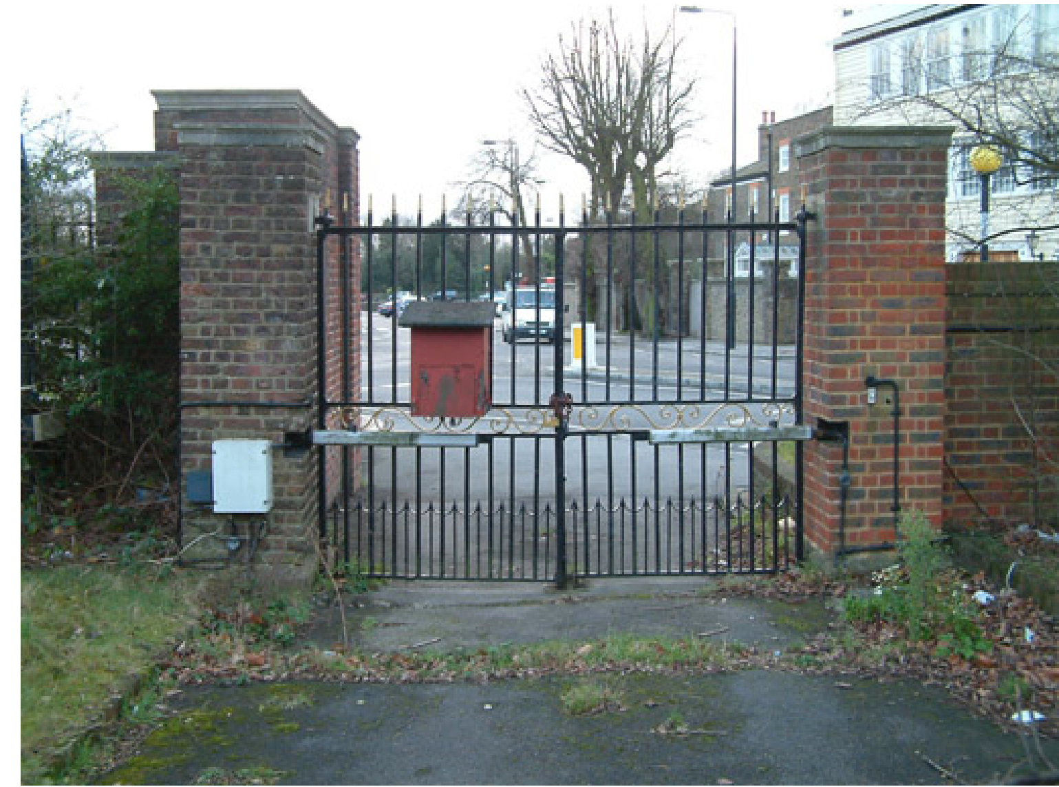
Existing gates shown from the forecourt of Heath House Pier 1 (right hand side of photograph) to be demolished and rebuilt to match Pier 2 (left hand side of photograph) to be retained and protected during the works
