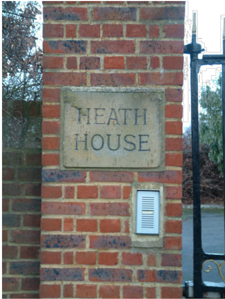
Detail of existing Pier 1 to be demolished and rebuilt to match Pier 2, existing gates removed and carefully stored for later rehanging
