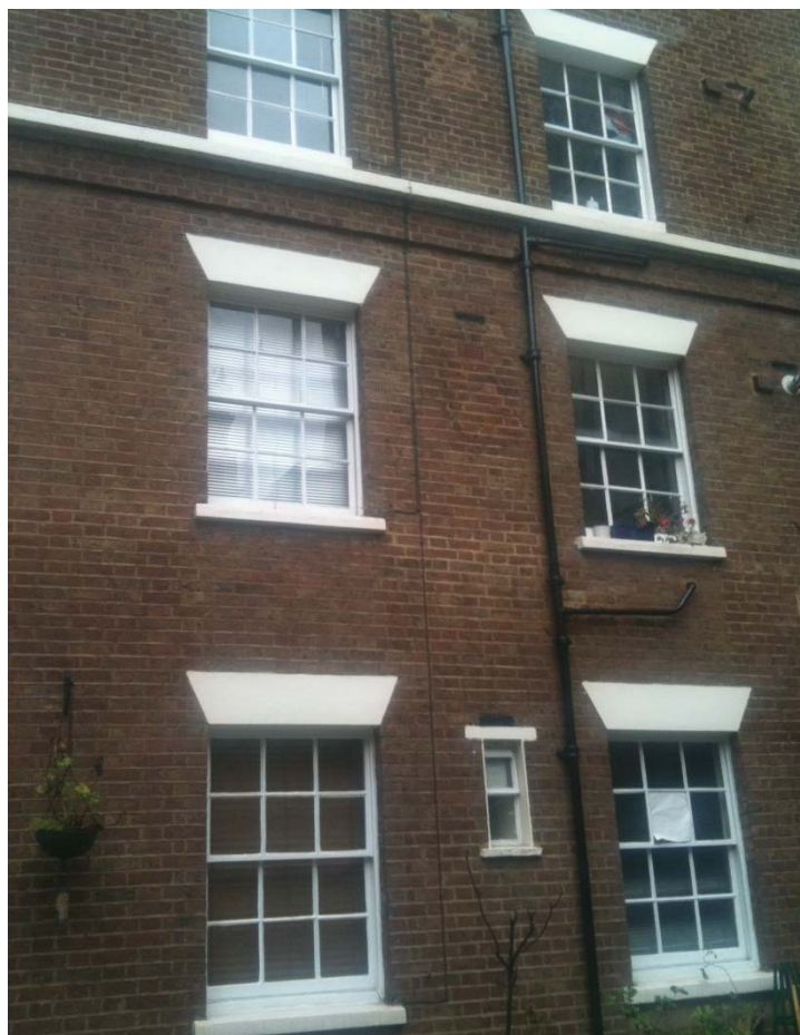
Photograph 14 – Existing cabling to be replaced at South east facing elevation of Courtyard
