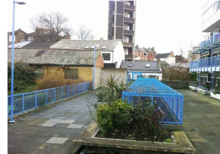
View of site from adjoining flats property
