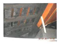
Although not visible from ground level, the extensive damp ingress from the roof coverings, together with the age of them would suggest they are at the end of their life. Allow for replacement of the roof coverings.
