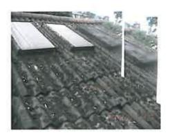
The ridge line of the main roof is very uneven and the clay ridge tiles will require taking off and rebedding as part of the roof replacement works.
