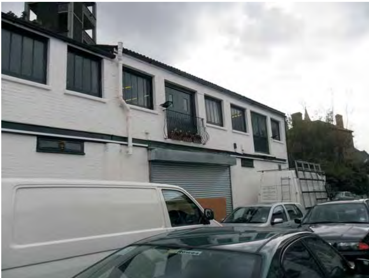
Plate 4 South facing photograph of late 19th century workshop, currently in use as a piano warehouse
