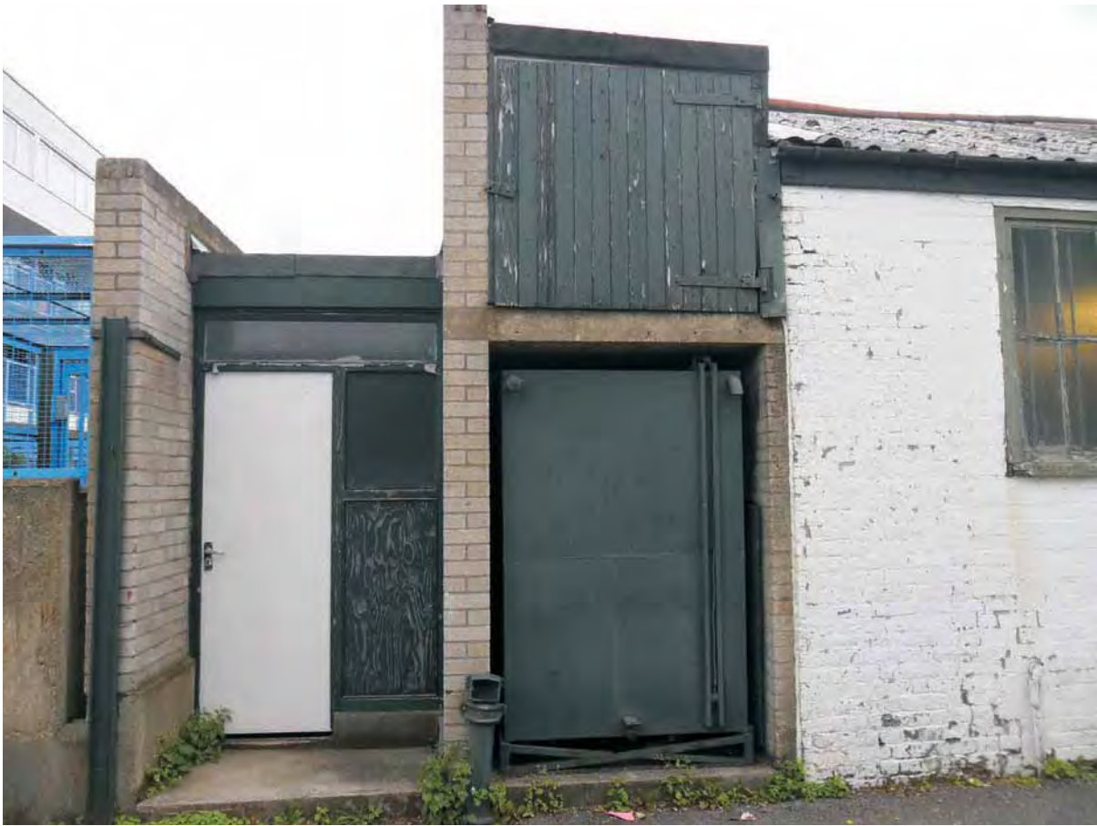
Plate 5 North west facing photograph of modern extension abutting the joiners workshop
