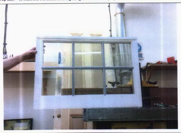
Bottom sash – to illustrate the sections and glazing bars - note the proportions of the windows will be as existing.
