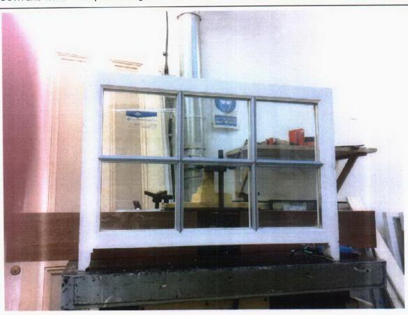
Top sash – to illustrate the sections and glazing bars - note the proportions of the windows will be as existing.
