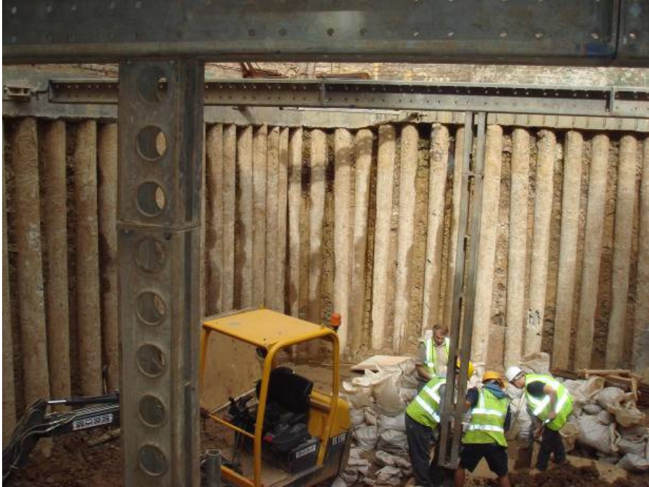
Figure 1- Contiguous piled wall at a similar project at Chepstow Villas W11. Note bracing props in picture to resist lateral forces until basement box structure has been cast.
