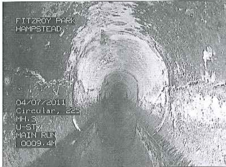
Photo: 4_11a, Tape No.: 5110, 00:01:48 9.4m, Deformed drain/sewer 10 %
