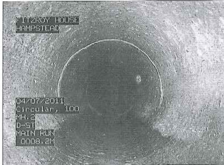
Photo: 37_7a, Tape No.: 5110, 00:02:11 5.2m, Fracture Circumferential from 12 to 12 o'clock
