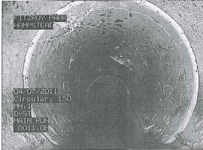
Photo: 1_12a, Tape No.: 5110, 00:03:47 11m, Crack Circumferential at joint from 10 to 03 o'clock
