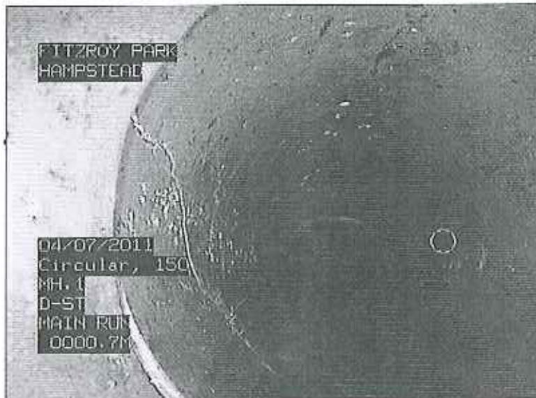
Photo: 1_5a, Tape No.: 5110, 00:00:42 0.7m, Circumferential Fracture at joint from 06 to 09 o'clock
