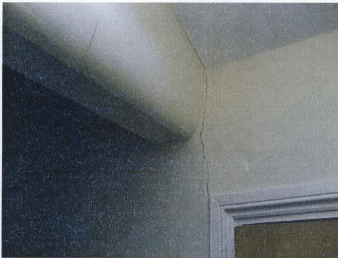
Cracking across dropped beam at junction of rear projection
