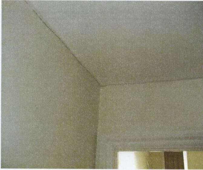
Wall-Ceiling Separation within Rear Bedroom
