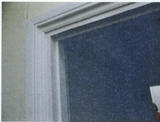
Wall-Ceiling Separation within Rear Bathroom
