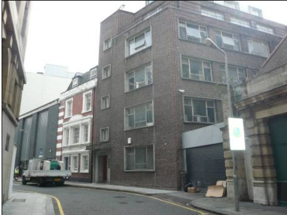
Photo 1: View looking south east across the existing site from Fisher Street (the tall brown brick building and red Georgian style building are to be demolished).
