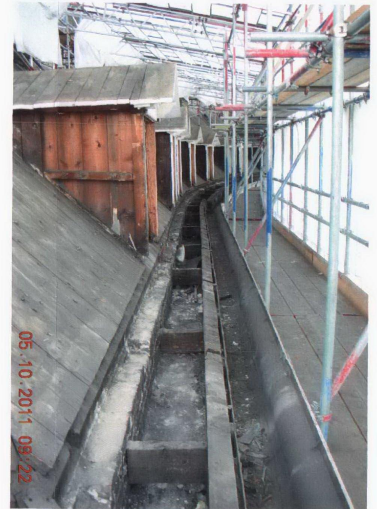
Detail 02 Existing Cornice Structure Opened Up
