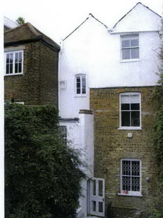
VIEW OF BRICKWORKS AND WHITE PAINTED RENDER
