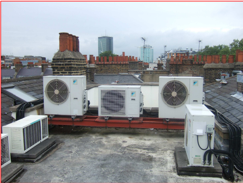
EXISTING CONDENSER MOUNTED ON EXISTING STEELS TO REMAIN.
