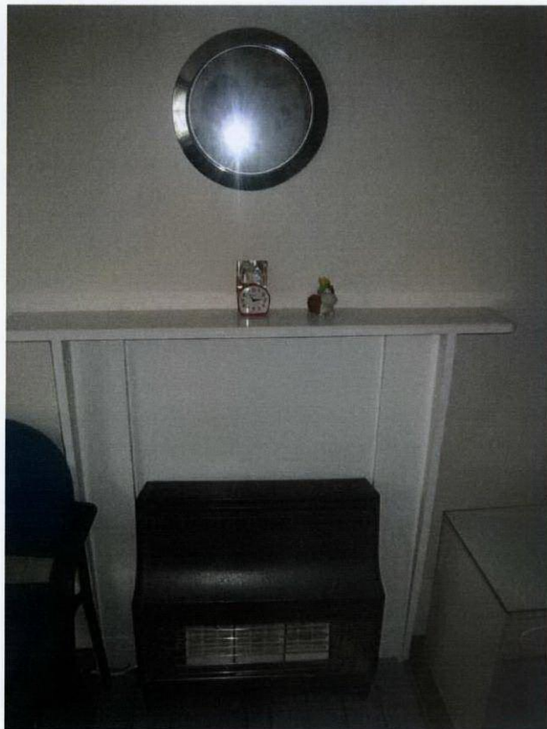
Master Ensuite rF.02 - Existing Fireplace Hearth and surround to be removed
