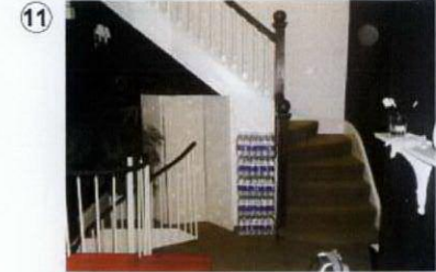
Contemporary stairs to first floor level and modern spiral stairs to basement to be removed
