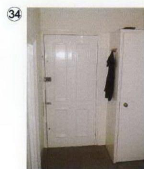
Recent lobby partition, door and cupboard at head of stair to be removed and existing door to T2 to be blocked up
