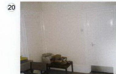
Contemporary doorway to be blocked up & possible original doorway to landing reinstated
