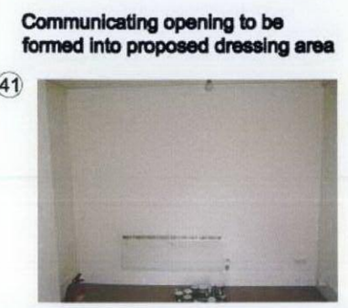
Partition and Nib to be removed to form bedroom, en-suite & dressing area
