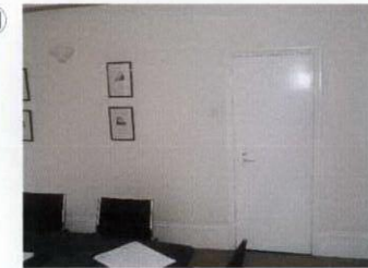
Later partition and door to be removed to return room to original proportions
