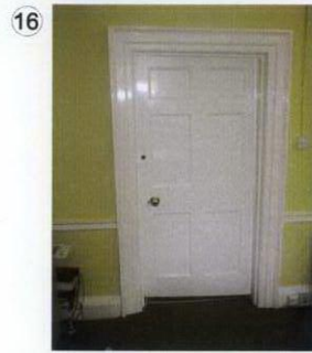
Existing doorway to be blocked up to form bathroom area. Door leaf salvaged for reuse with reinstated door
