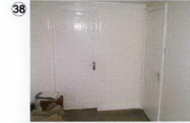
Contemporary communicating door to be removed. Opening to remain
