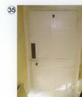
Original door frame and architraves retained
