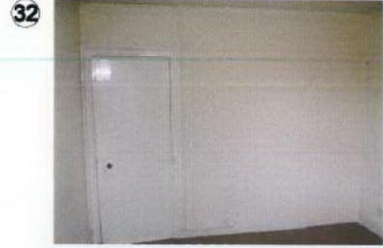
Possible original panelled partition retained. Door leaf removed
