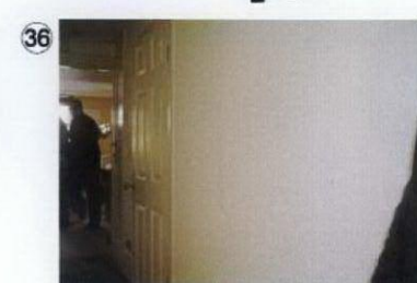
Partitions forming shower room/WC to be removed
