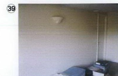
Later partition & door to be removed to return room to original proportions
