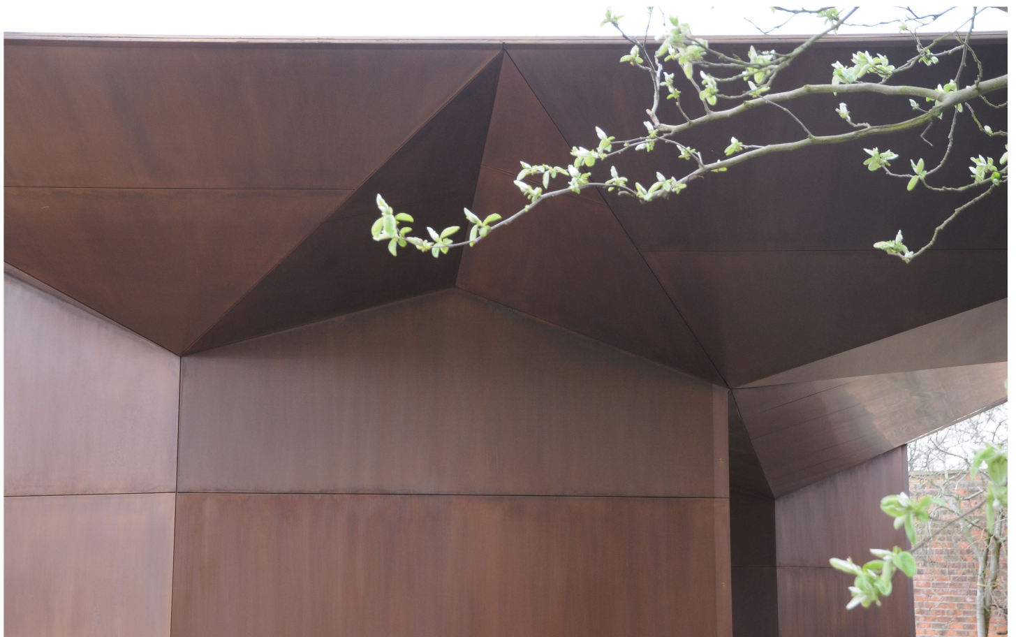
Patinated Gilded Metal Canopy and Cladding
