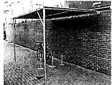
the wall there will be 4x scaffold poles bolted into the ground (concrete) and the roof to be of plastic black corrugated sheet.
