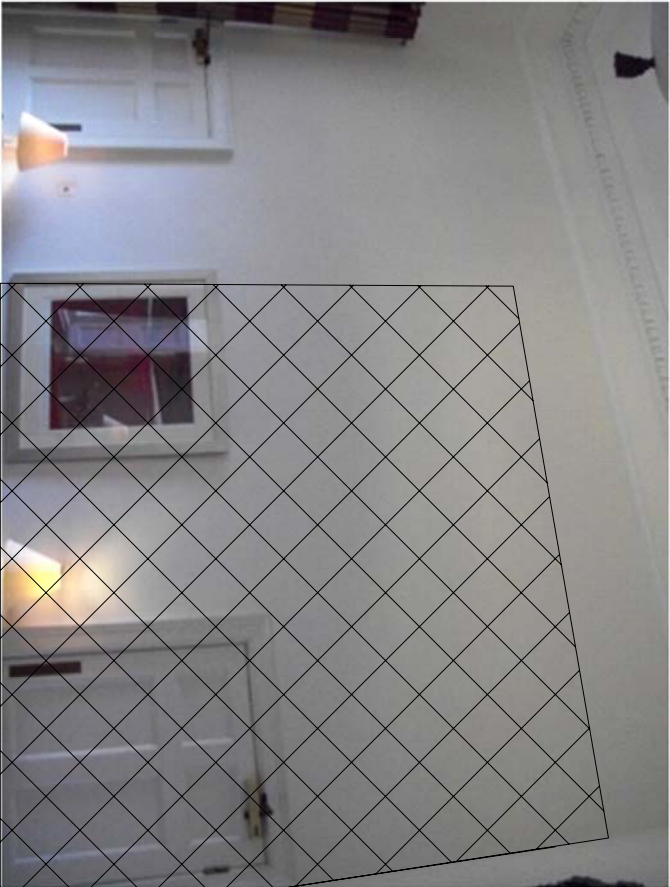
IMAGE SHOWING SECTION OF WALL TO CREATE OPENING (VIEW FROM WAITING ROOM)
