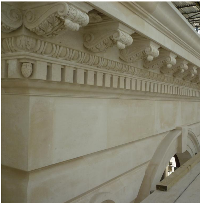
Photo 3: Cornice and stonework
