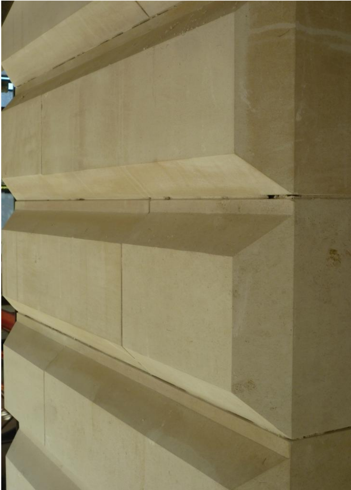
Photo 4: Facing stonework detail
