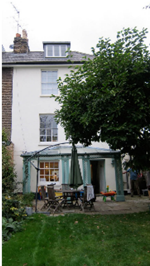
6. Existing 1990's Glazed porch
