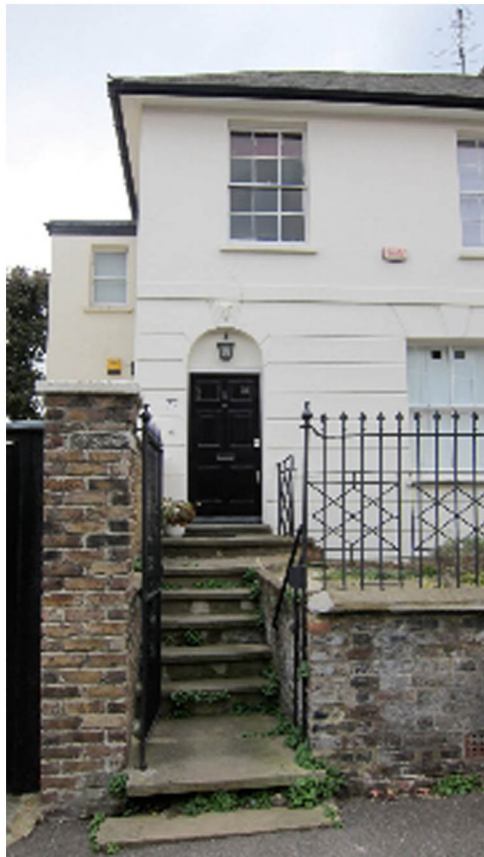
1. No. 37 Downshire Hill
