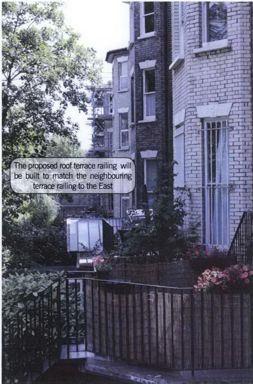
Views to the East at the rear of the building.
