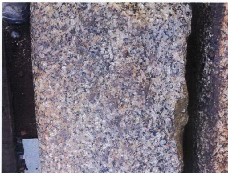
Image 10: Detail Image of site won granite kerbs
