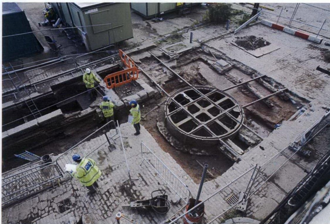
Image 3: The relationship of Crane base 1 and Turntable B
