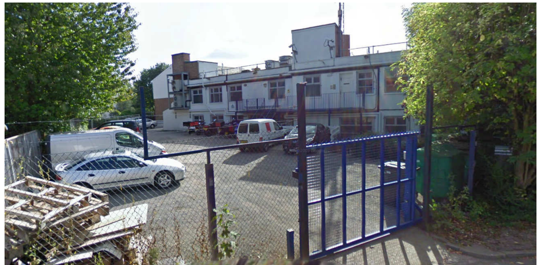
Rear Site Access
