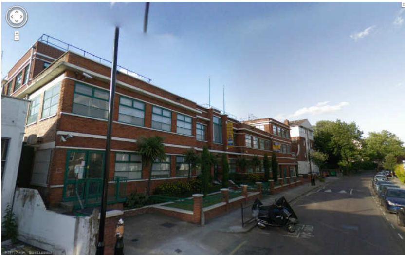
Maygrove Road Frontage
