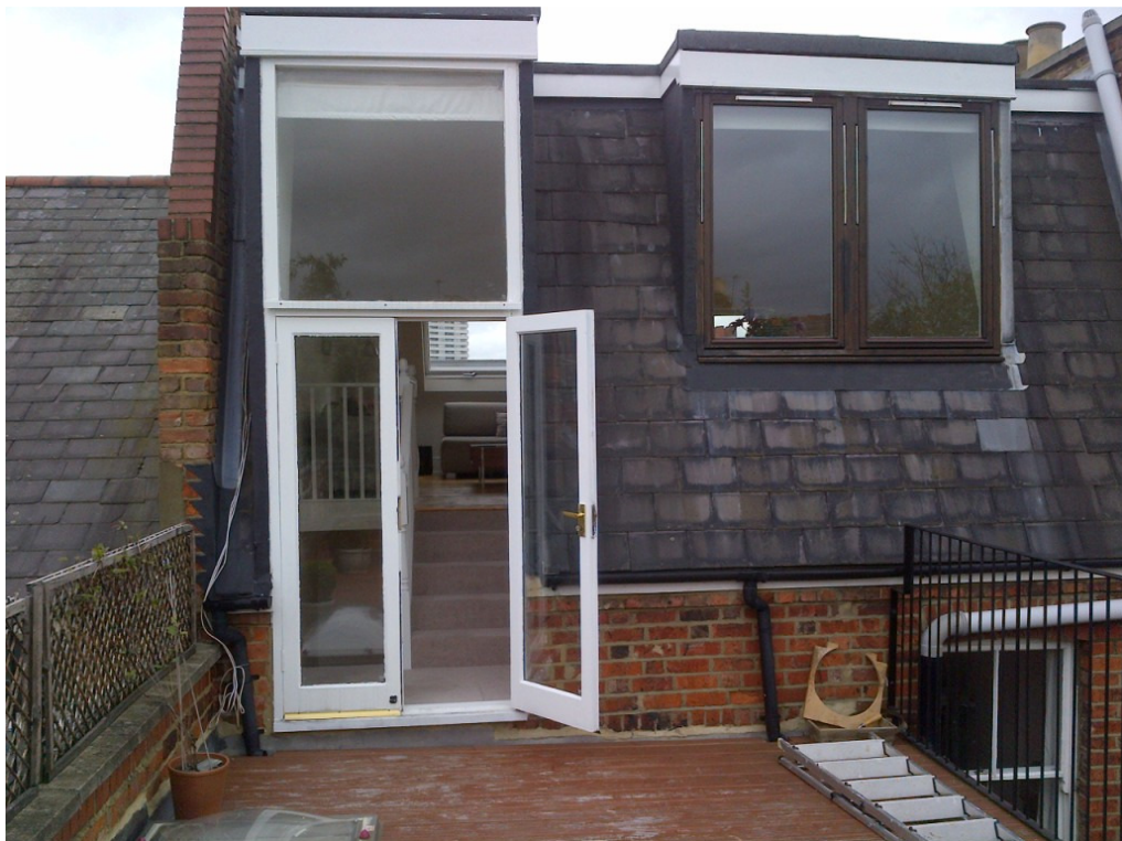
Rear Elevation .Pic01
