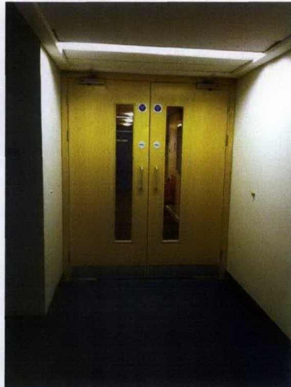
8: Existing suspended ceiling to be removed & new plasterboard ceiling to be installed
