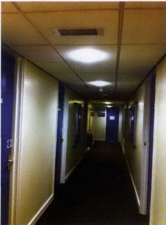
8: Existing suspended ceiling to be removed & new plasterboard ceiling to be installed
