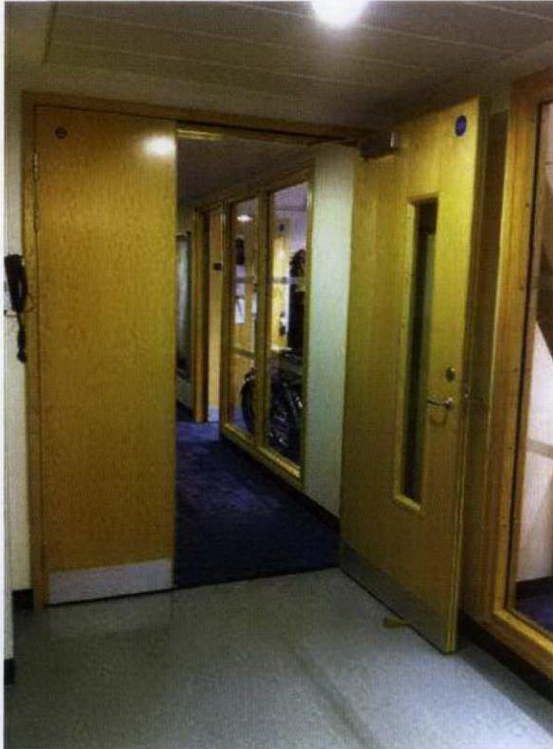
7: Previous application finish on 5 th floor 26 Bedford Way. New hardwood doors with veneer finish as above, to be installed on the 4 th floor with full height glass partitions for natural light.
