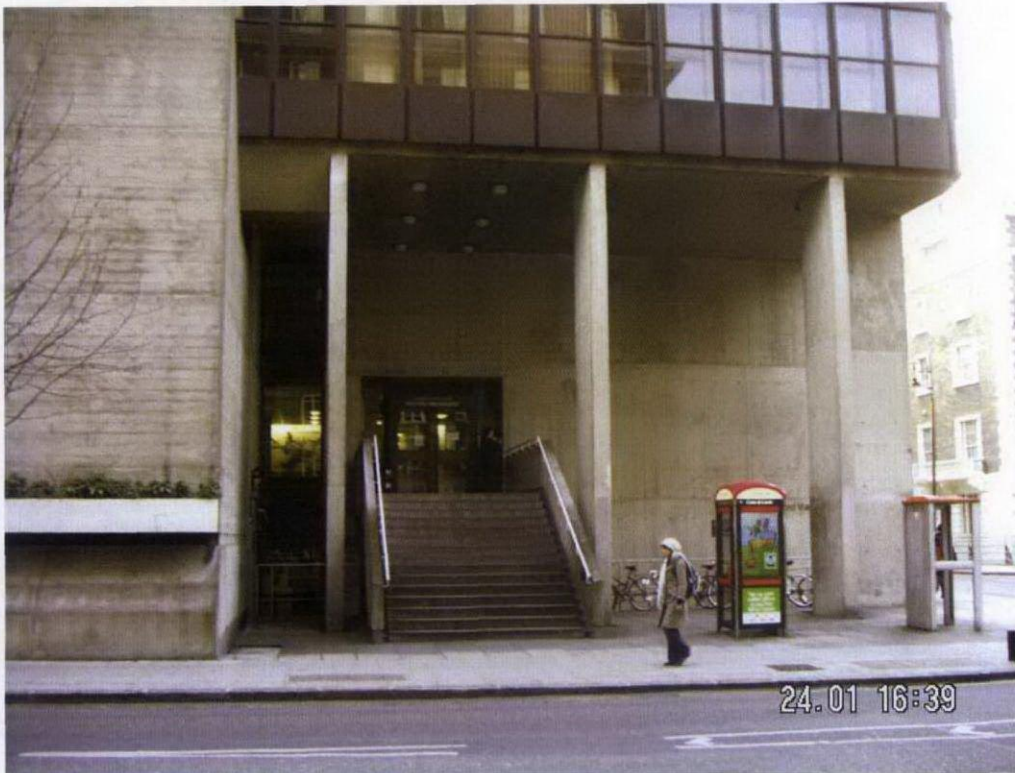
1: Main Entrance up to Ground Floor from Street level to 26 Bedford Way (East elevation)
