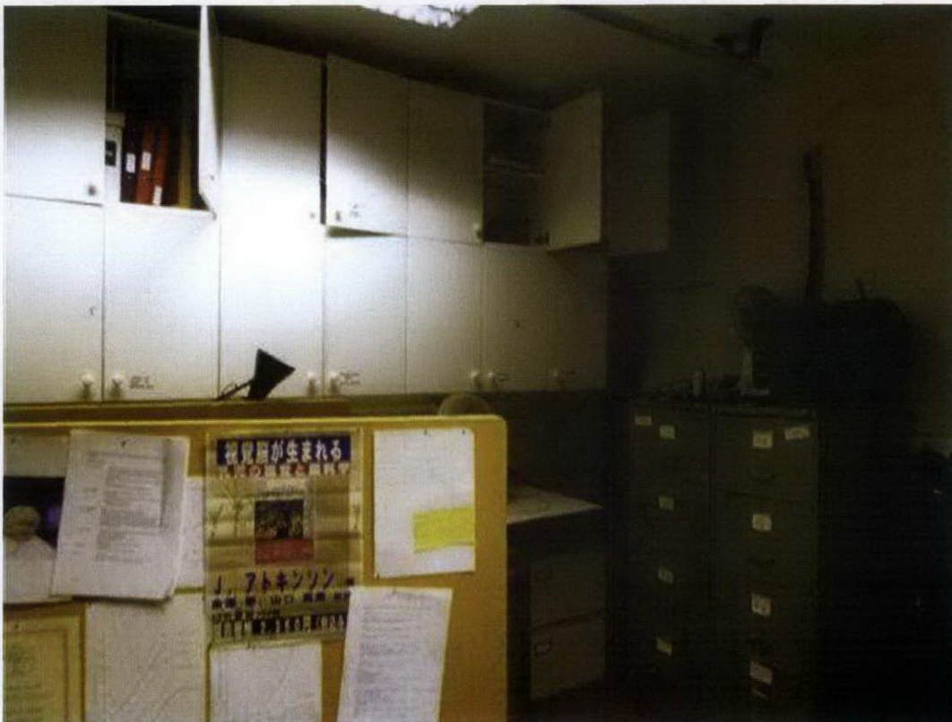
6: Strip out of all existing wall mounted cupboards, fixtures & fittings.
