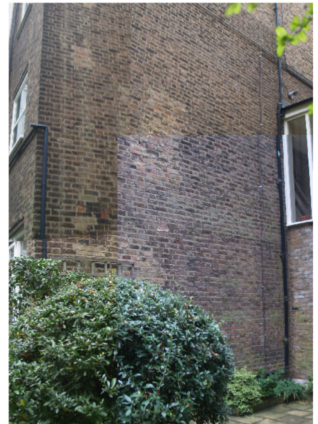
EXISTING WEST ELEVATION CLOSE UP
