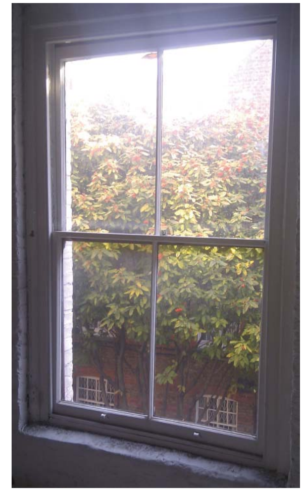
Image of existing window - Proposed timber framed clear double glazed units to match.
