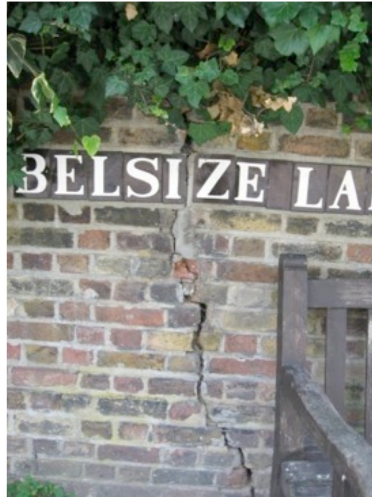
View2: Boundary wall condition - Cracking caused by 2 no London Planes – now removed with consent
