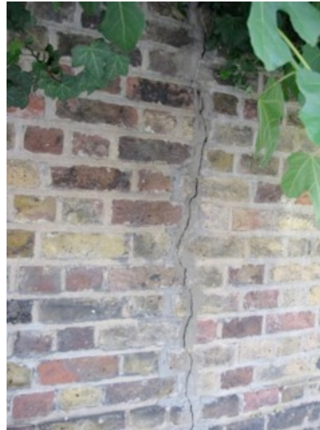
General View. Boundary wall condition- Cracking and split bricks
