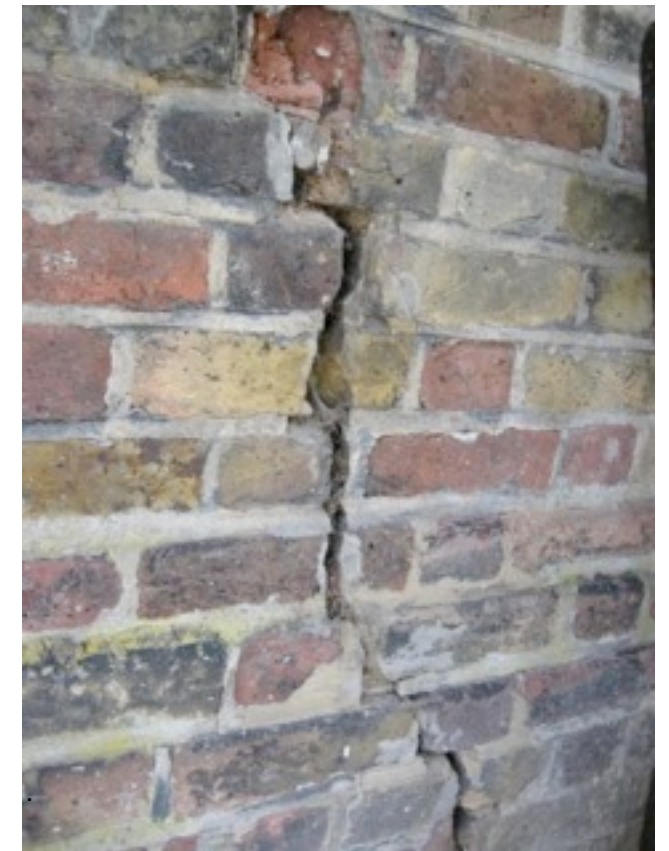
General View. Boundary wall condition Cracking and split bricks
