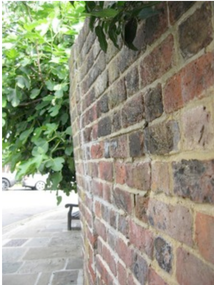
View1: Boundary wall condition - Possibility of collapse due to foundations being undermined
