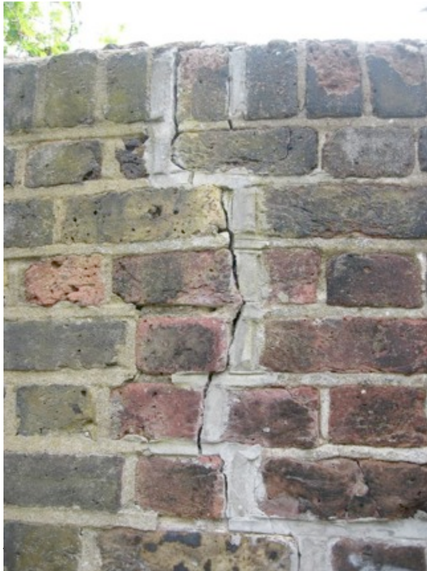
General View. Boundary wall condition –cracks repaired with excessive pointing
