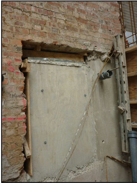
UNDERPINNING TO A PARTY WALL
