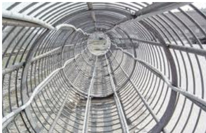
Energy pile before installation
