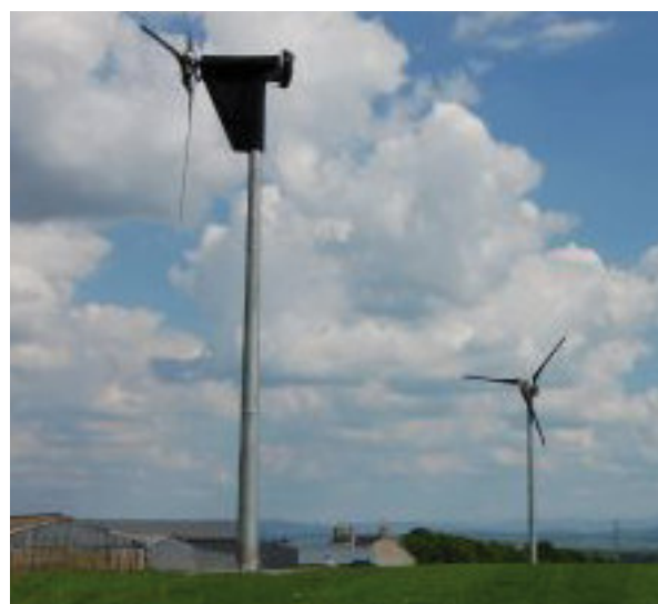
Two 12kW Proven Wind turbines
