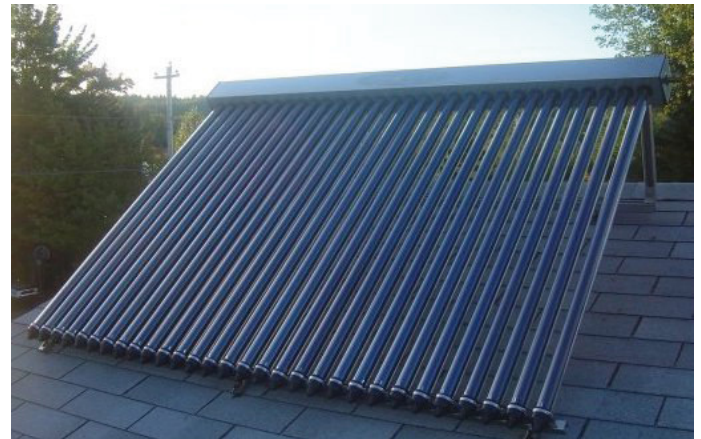
Evacuated Shell and Tube Solar Thermal Panel
