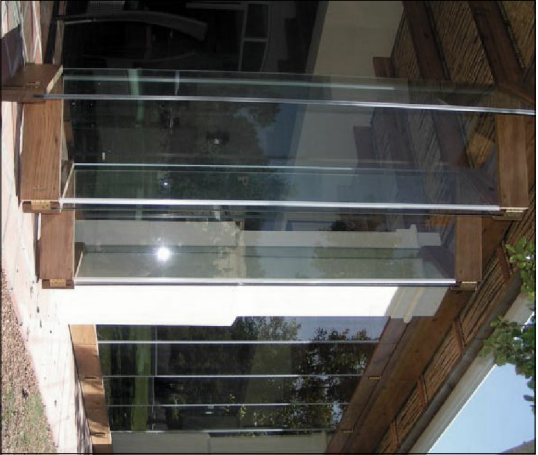
Folding frameless door in 4 sections to both extensions to allow full opening of aperture
