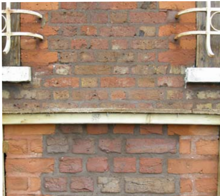
Existing brickwork (above) with Sample panel (below)
