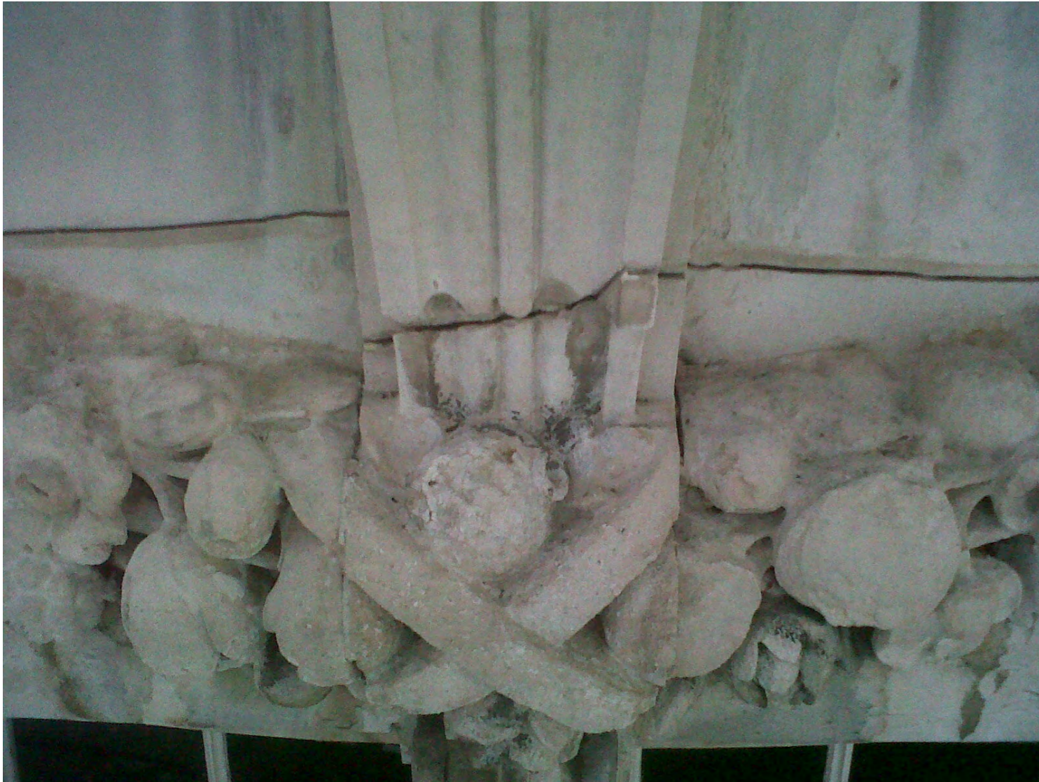
PH01 - Horizontal crack to central bay of 3rd floor cornice to front elevation
