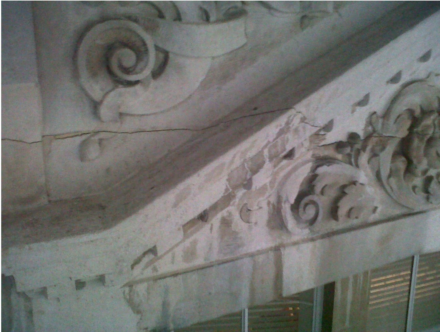
PH05 - Horizontal crack to left hand bay of 3rd floor cornice to front elevation
