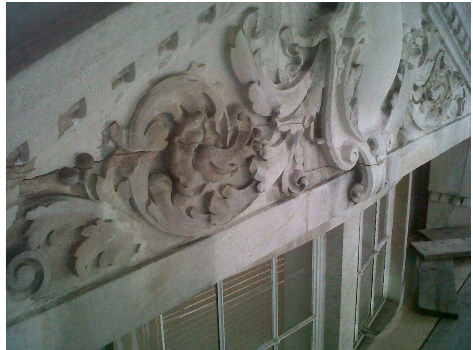
PH06 - Horizontal crack to left hand bay of 3rd floor cornice to front elevation
