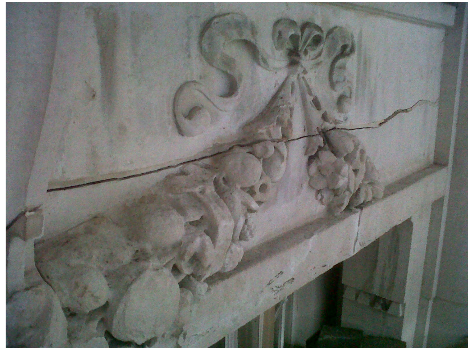
PH02 - Horizontal crack to central bay of 3rd floor cornice to front elevation
