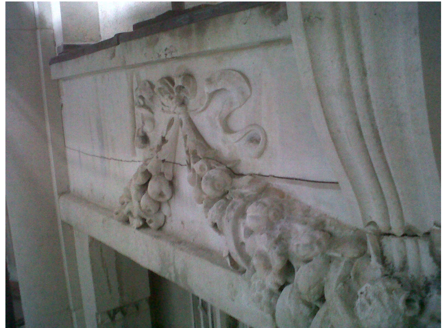
PH04 - Horizontal crack to central bay of 3rd floor cornice to front elevation
