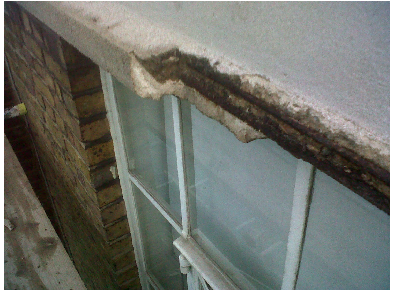
PH08 - Spalling concrete lintel to rear elevation
