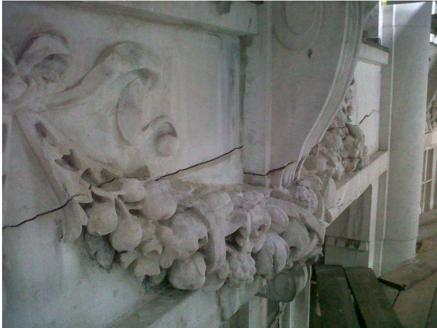
PH03 - Horizontal crack to central bay of 3rd floor cornice to front elevation
