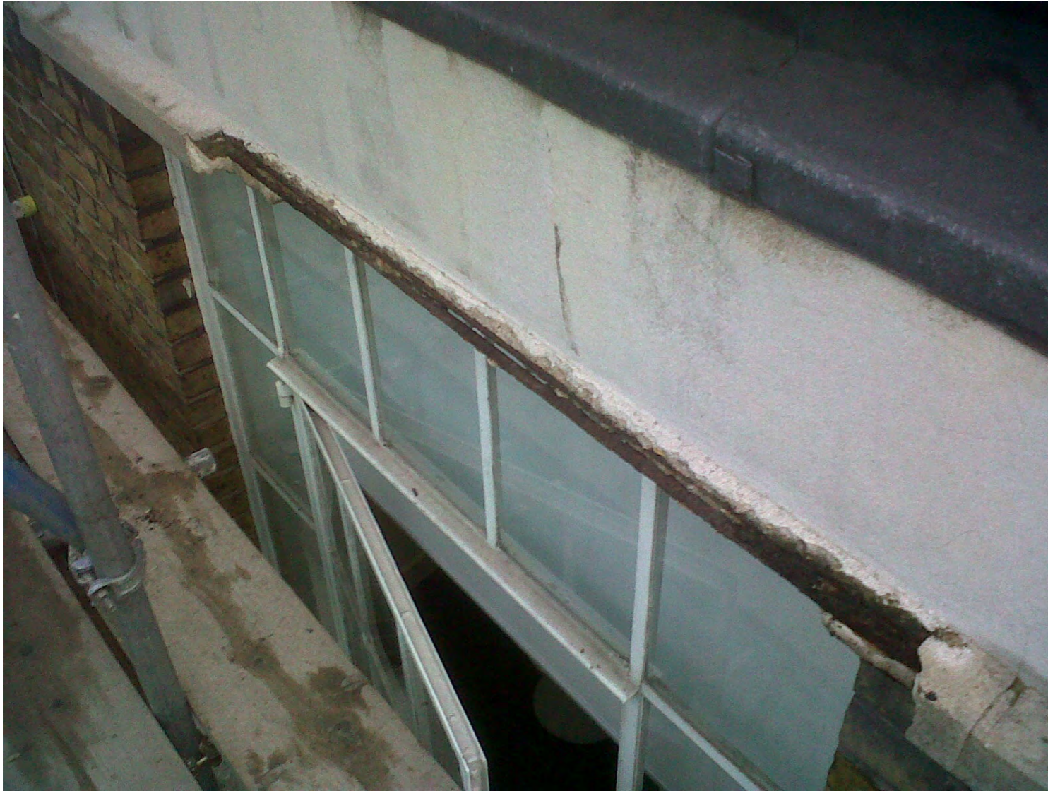
PH07 - Spalling concrete lintel to rear elevation
