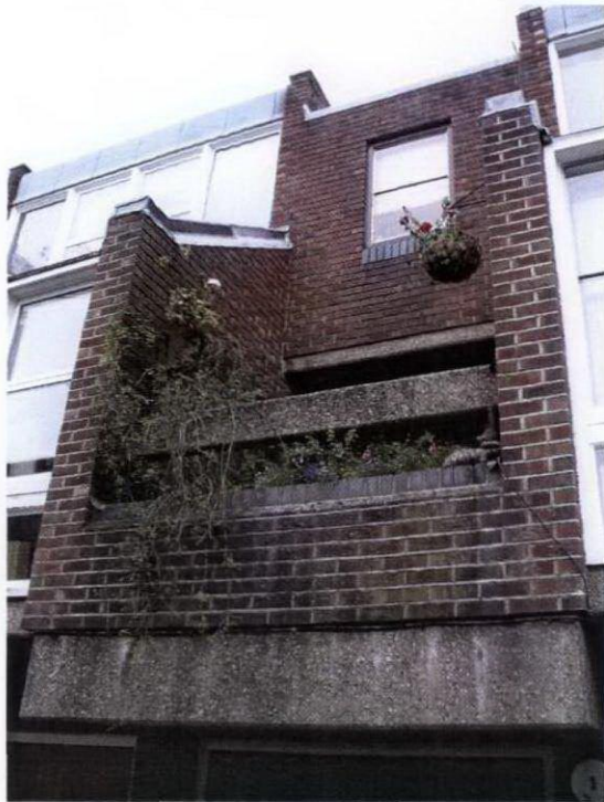
3 Lakis Close existing balcony
