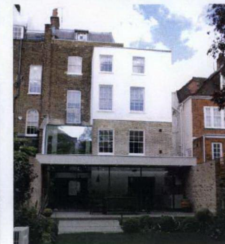
Hamilton Terrace NW8 - Extension & modernisation of grade II listed terrace house
