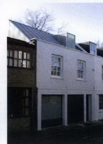
Kingsdown Street, NW1 - Partial rebuild & extension to 1930s 4 conservation area new house
