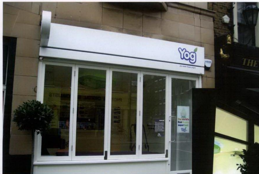
Frontage - prior to alteration
