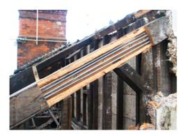
Repair of fire damage to rafter of principle roof truss.
