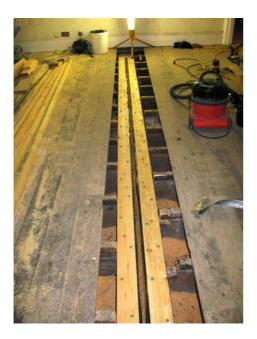
Reinforcement bars inserted into slot and bonded into position with epoxy resin.
