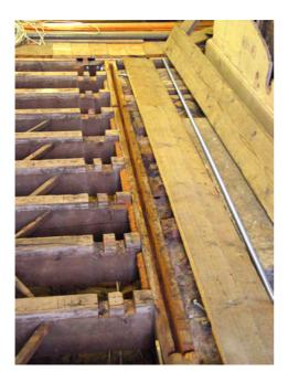
Reinforcement of hearth trimmer using slot method without damage to joist joints
