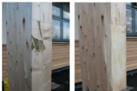
Repair and replacement of damaged or decayed structural members and frame components.
