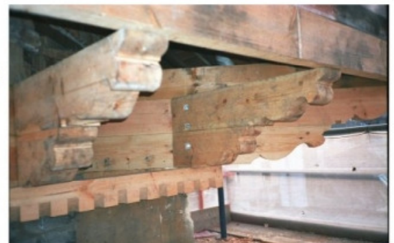
Repair and replacement of damaged or decayed structural members and frame components.
