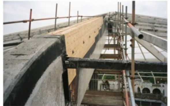
Erection and repair of laminated timber frame structures.
