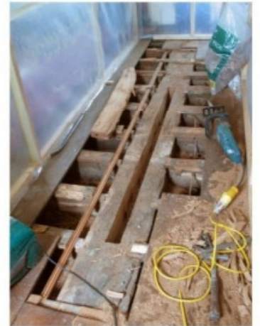
Repair and strengthening of structural timber components using reinforced epoxy resin techniques
