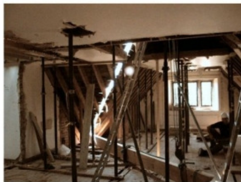
Repair to listed timber frame buildings using traditional timber replacement and jointing methods.
