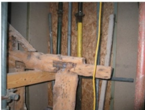
Repair and strengthening of structural timber components using reinforced epoxy resin techniques
